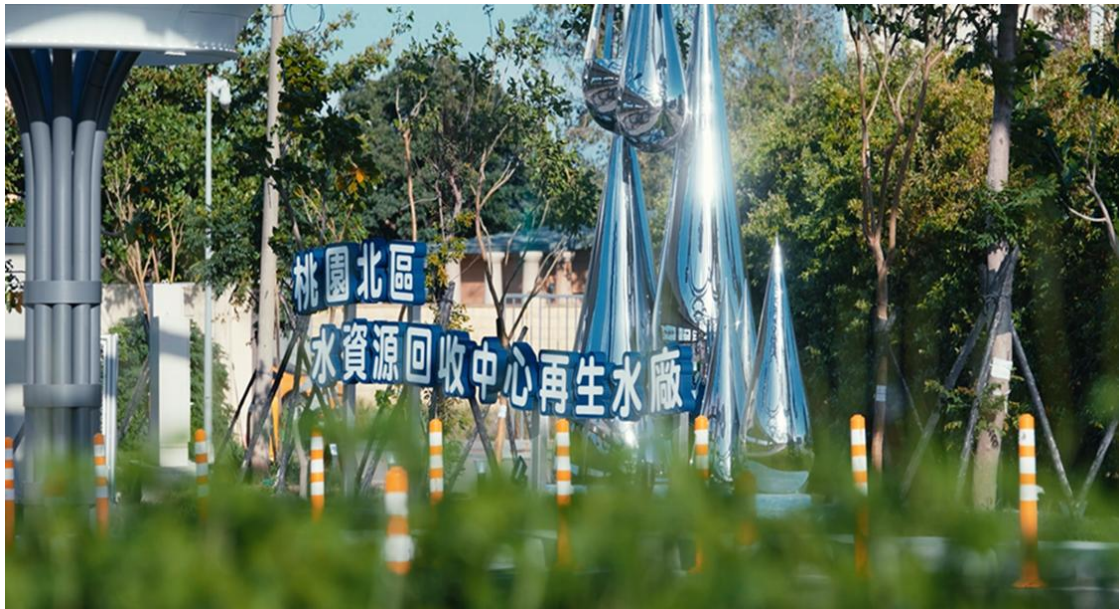
Bao Ding Reclaimed Water- Taoyuan North District Reclaimed Water Center, ESG Park
